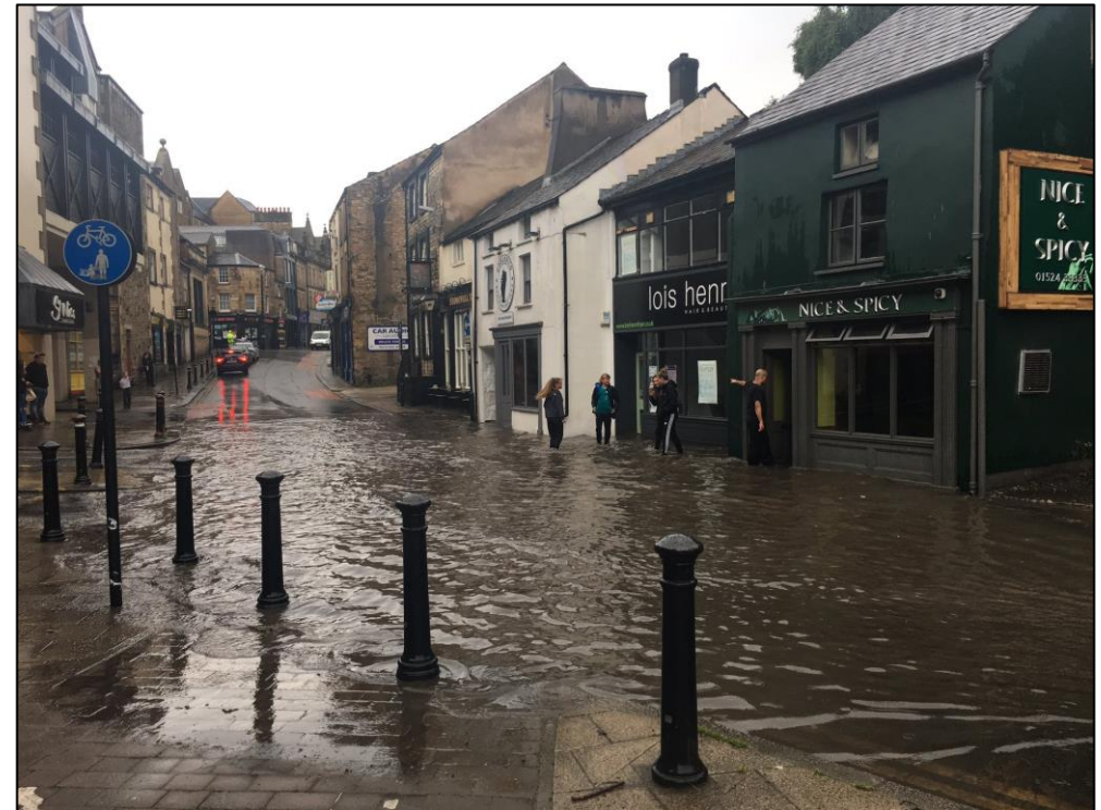
Figure 3.12: Surface water flooding Church Street – July 2017
